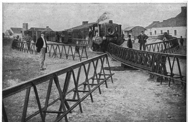
THE BEHR MONO-RAIL BETWEEN LISTOWEL AND BALLYBUNION, IN KERRY, IRELAND
